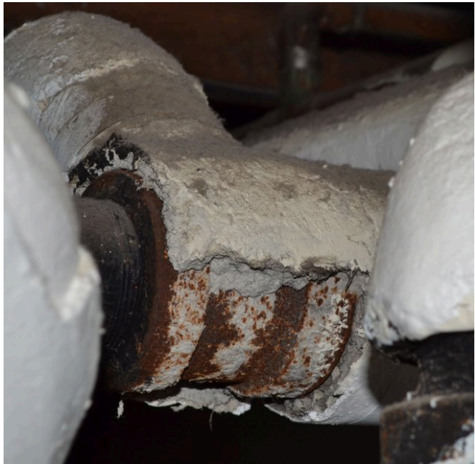
Asbestos pipe wrap (joint partially removed)
